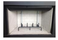
The installation is now complete. With the EPA Qualified Emission Control Device in place, the wood burning fireplace is now EPA Phase II Qualified and ready for efficient catalytic operation. The homeowner can display the EPA Hangtag that officially designates the wood burning fireplace as an EPA Phase II Qualified unit. When using the fireplace for the first time after installation of the emission control system, insure that you follow the **SAFETY WARNING** below:
